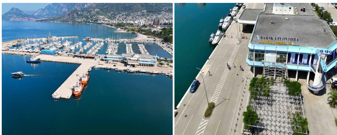
Photos 6-7. Passenger Terminal of the Port of Bar
