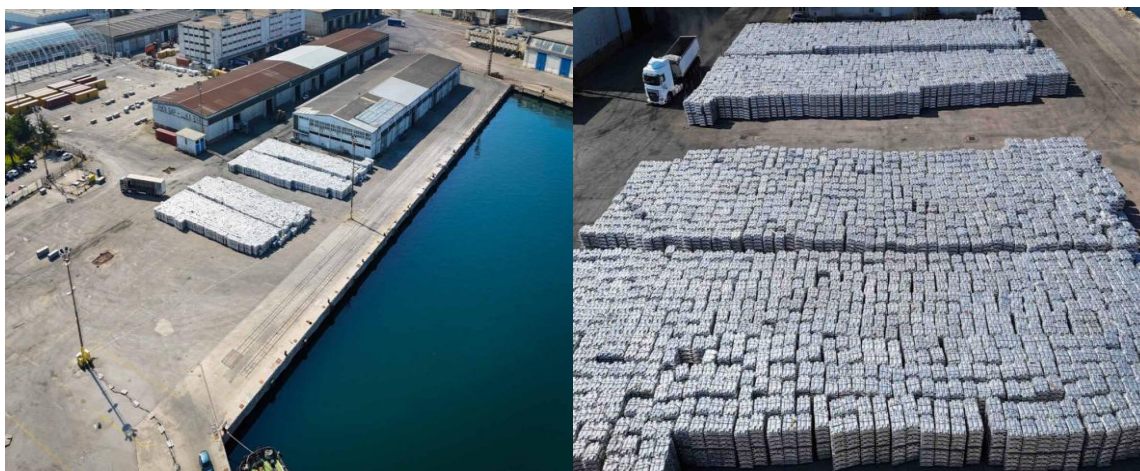
Photos 4-5. RO-RO, General Cargo, and Container Terminal
