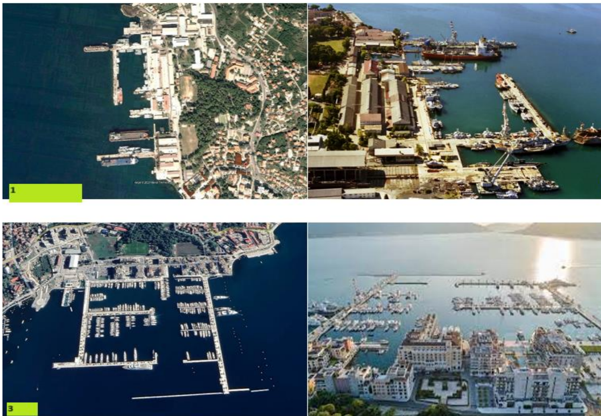
Figure 2. Naval Technical Overhaul Institute "Sava Kovačević" (1,2) and the current marina and nautical resort Porto Montenegro (3,4).
